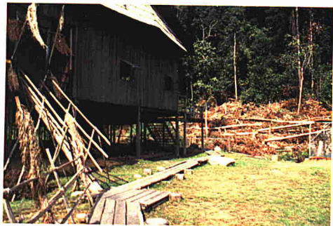
Bottom: An Orang Ulu longhouse built out of ironwood. This wood is extremely heavy and hard.
